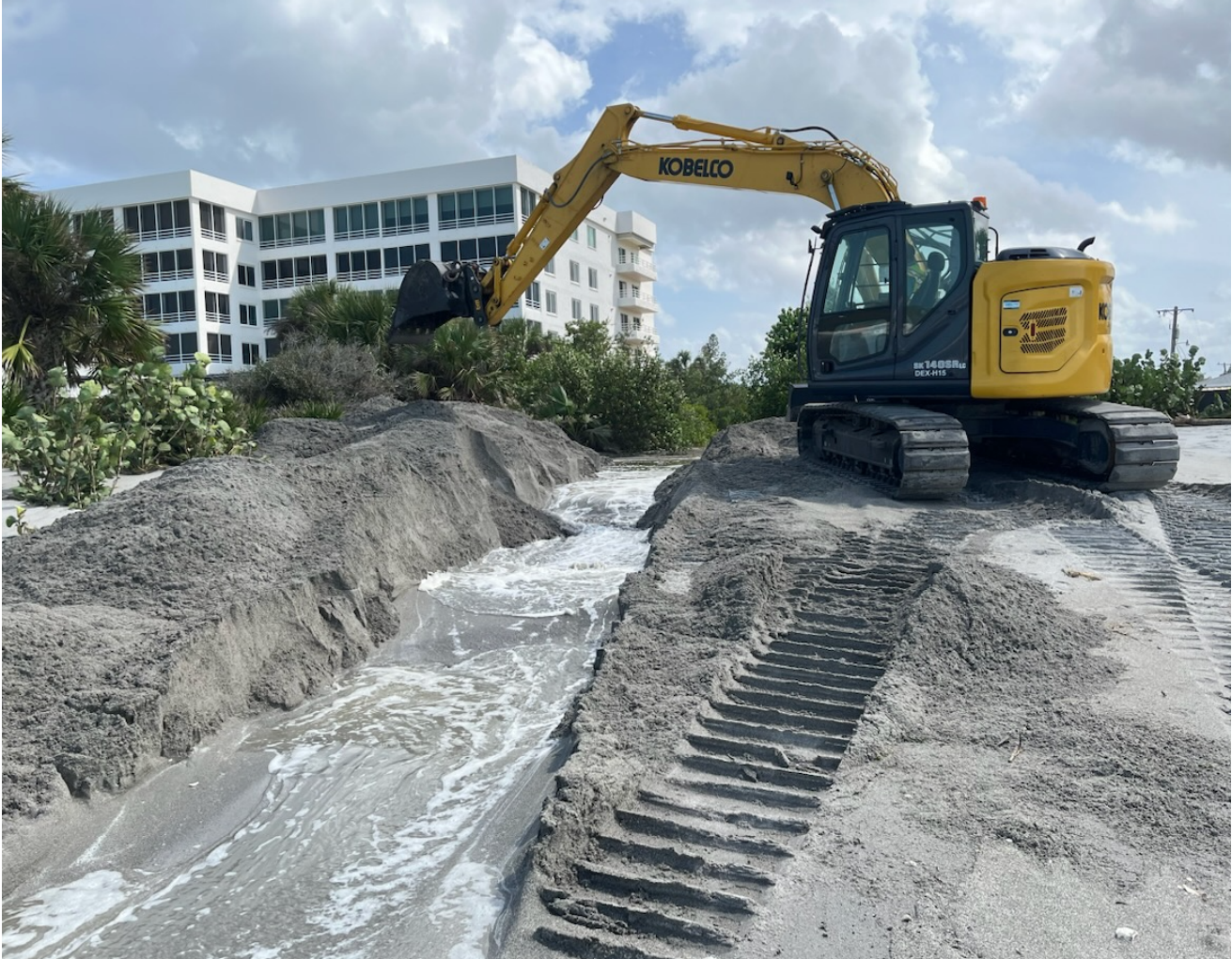
A city emergency worker “unplugs the ditch” Friday afternoon, draining the Golden Beach floodwaters like a bathtub.
