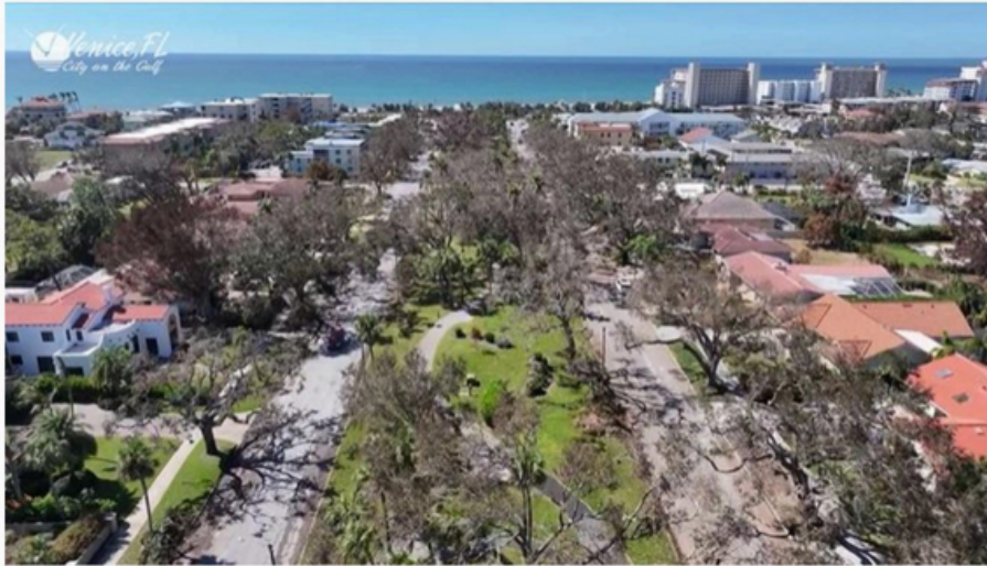
At left, an aerial photo of Heritage Park on West Venice Ave. after Hurricane Milton shows trees with extensive wind burn.
