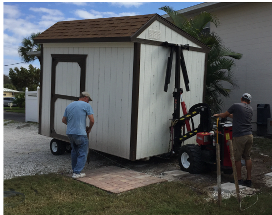
Moving the new shed into place
