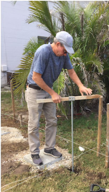
John sets a hurricane anchor
