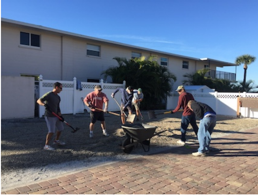
Loading the shells by shovel and distributing by wheelbarrow:
